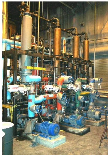
Physical installation of the hot oil system.
